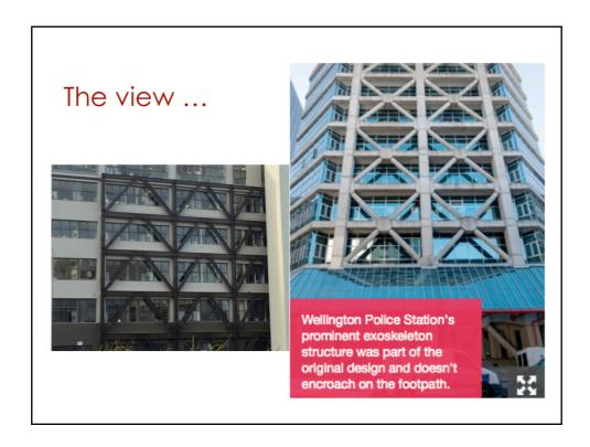
One method of strengthening is an exoskeleton. However, this will usually not markedly enhance a building's appearance. An architect may be able to design an exoskeleton that has less negative impact on the building that an engineer can.
